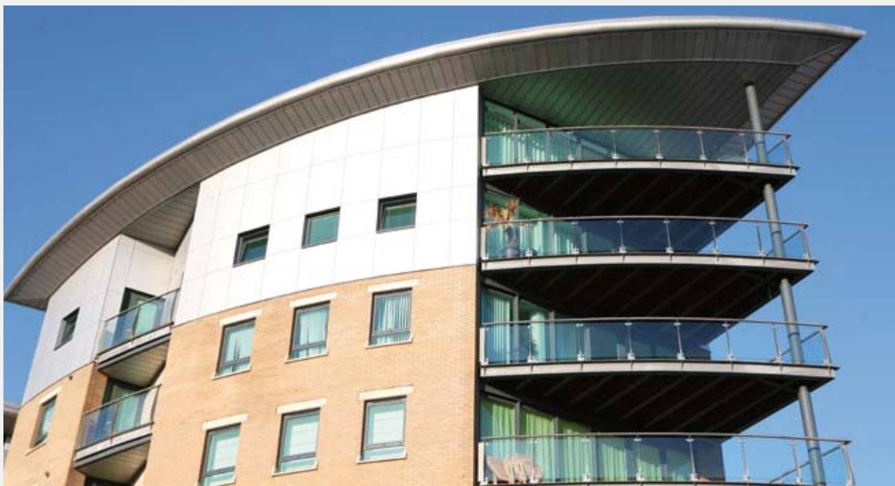
Outdoor building facade made of compact laminates produced with solid colour papers and printed designs.
