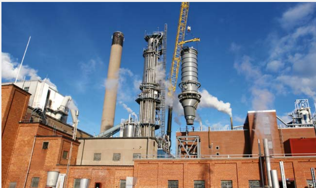
Installation of the pre-steaming vessel in Aspa Bruk.
